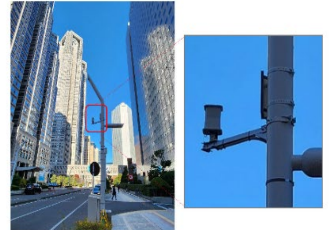
Repeater Installation in Nishi-Shinjuku Area
